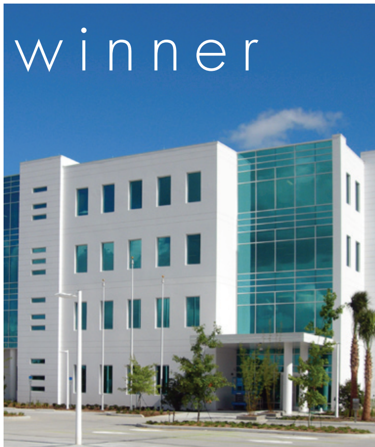
Toho Water Authority Headquarters Kissimmee, FL
